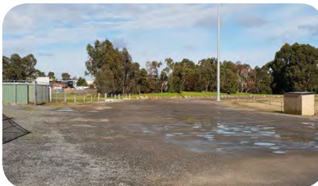
Unmarked gravel car parking around oval with pot holes and no line marking
