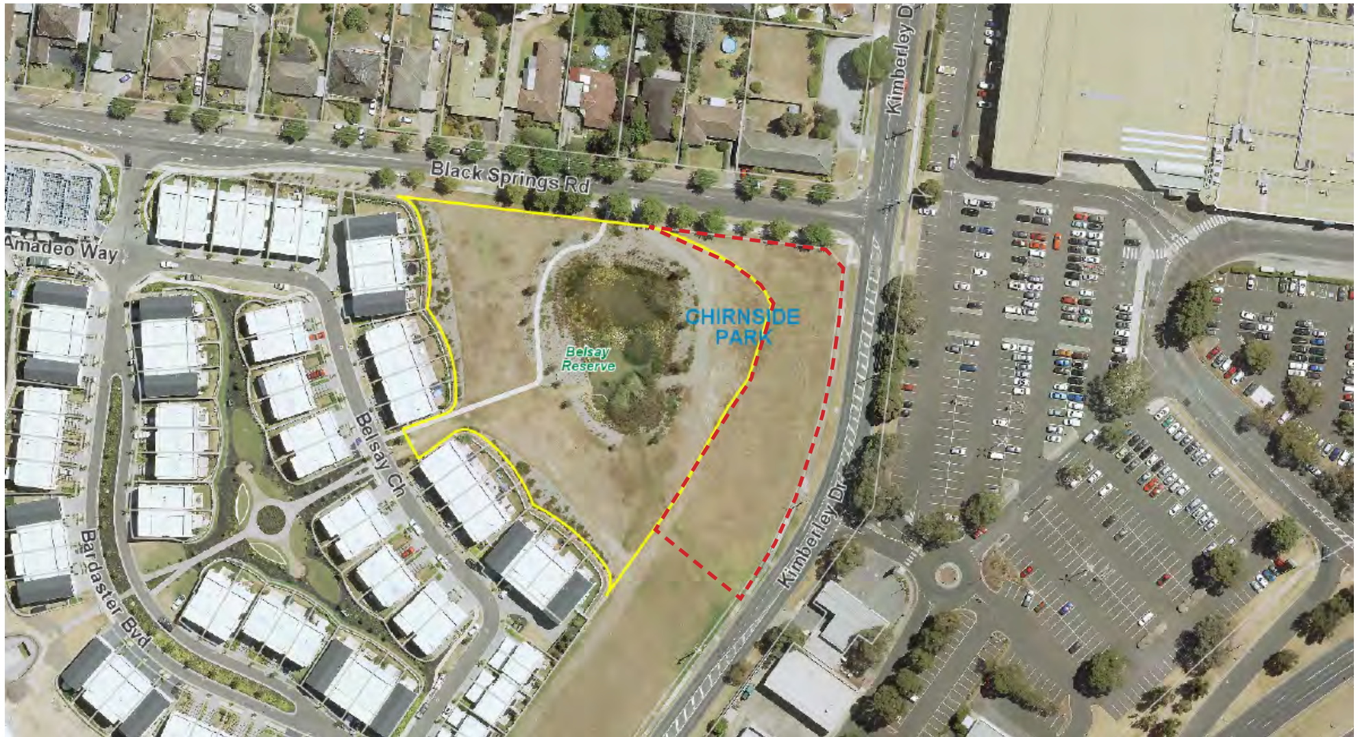
Figure 2 - The extent of the site area to be developed includes the area within the yellow line and the red dashed area (recently purchased by Council).
