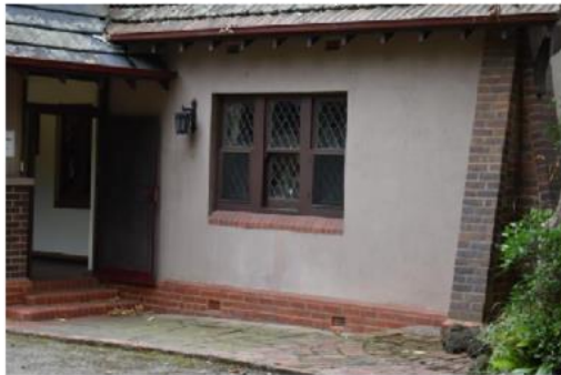
Detail view of ground floor fenestration, brick window sill, and clinker brick corner buttress (source: Extent Heritage Pty Ltd, 2022).
