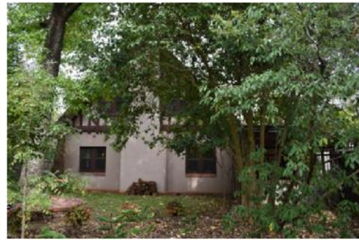
West facing view showing side elevation fenestration, half timber gables and chimney breast (source: Extent Heritage Pty Ltd, 2022).
