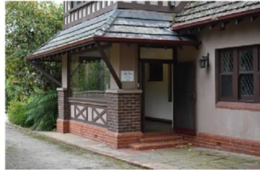
Detail view of entrance portico and awning (source: Extent Heritage Pty Ltd, 2022).
