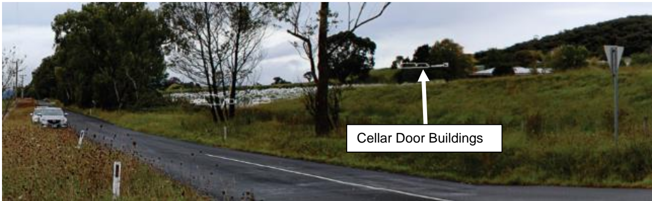
Figure 24 South-east facing view from intersection of Maddens Road and Briarty Road
