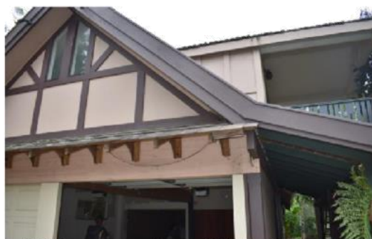
Detail view of upper floor addition, gable end and awning of garage (source: Extent Heritage Pty Ltd, 2022).
