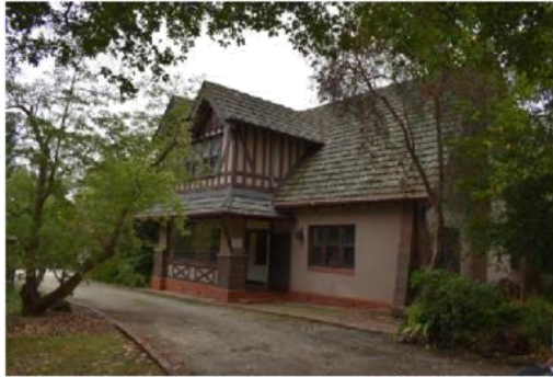
North-west facing view of main residence from driveway (source: Extent Heritage Pty Ltd, 2022).
