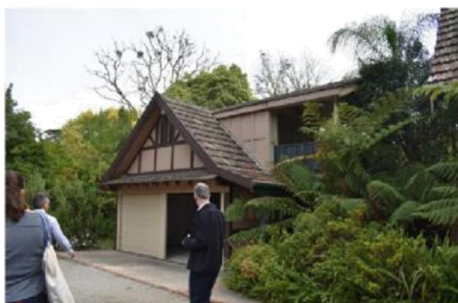
North-west facing view of garage (source: Extent Heritage Pty Ltd, 2022).
