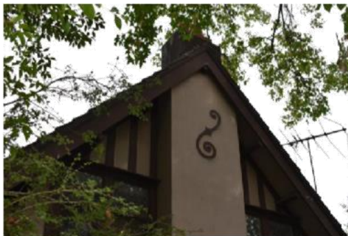
Detail view of S shaped wall tie and chimney breast (source: Extent Heritage Pty Ltd, 2022).
