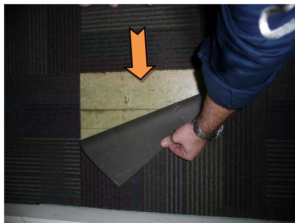
Photo 2. Main Building – ground floor call centre – under carpet tiles – assumed asbestos vinyl floor tiles.
