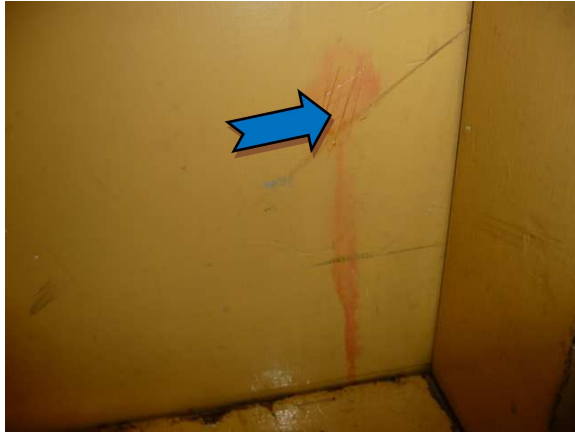
Photo 19. Main Building 1 st floor roof access point – doors and doorway – yellow lead-containing paint.
