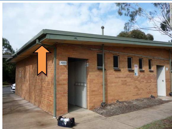
Photo 18. Contact Centre and Public Toilets – external eaves – asbestos cement. Sample 19952-001-009.
