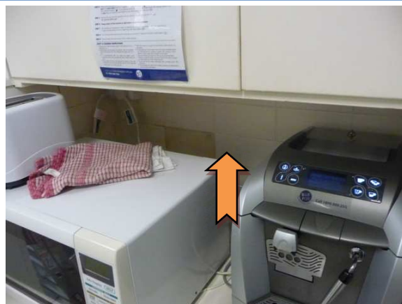
Photo 8. Main Building 1 st floor – kitchen – asbestos cement splash back behind ceramic tiles. Sample 19952-001-022.
