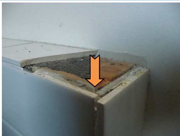
Photo 7. Main Building 1 st floor – male W.C. – asbestos cement lining behind ceramic tiles. Sample 19952-001-020.
