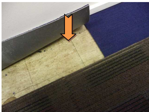
Photo 1. Main Building – ground level – under carpet tiles – asbestos vinyl floor tiles – Sample 19952-001-001A.
