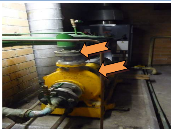
Photo 12. Main Building basement – Plant Area 1 – pump unit - assumed asbestos gaskets.
