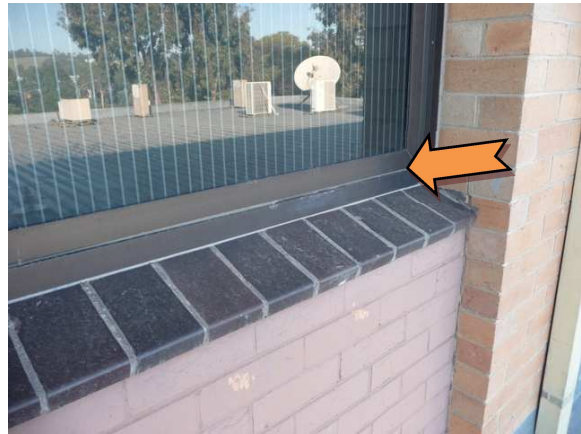
Photo 14. External roof area Main Building – windows throughout – asbestos-containing mastic – Sample 19952-002-002.
