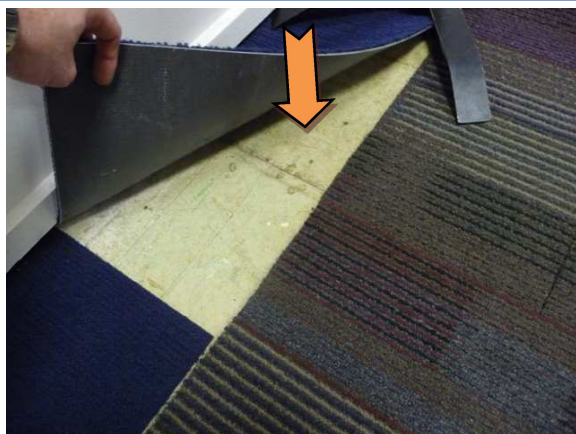
Photo 3. Main Building – Governance/CEO Area – under carpet tiles – asbestos vinyl wall tiles – Sample 19952-001-003A.
