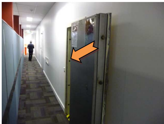
Photo 5. Main Building – ground floor – safe room 1 – assumed internal asbestos-containing fibre cement sheet.
