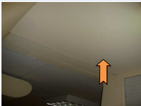
Photo 9. Main Building – basement corridor ceiling – asbestos cement. Sample 19952-001-024.
