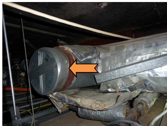
Photo 6. Main Building – Call Centre – asbestos mastic to joins in ductwork – Sample 19952-001-015.
