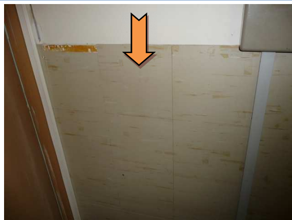
Photo 4. Main Building – IT/Comms room – walls – asbestos vinyl wall tiles – Sample 19952-001-0012A.
