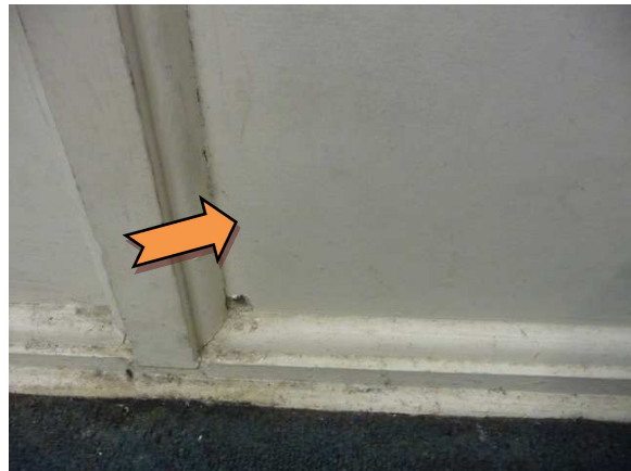
Photo 16. Contact Centre – east wall panels under windows – asbestos cement – Sample 19952-001-019.
