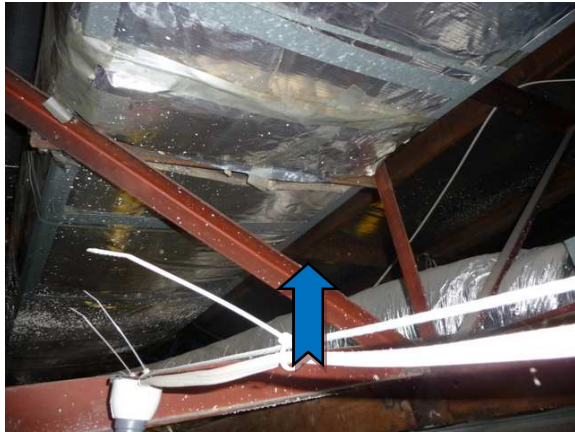
Photo 21. Main Building 1 st floor ceiling space throughout – suspected SMF insulation in fixed air conditioner ductwork.
