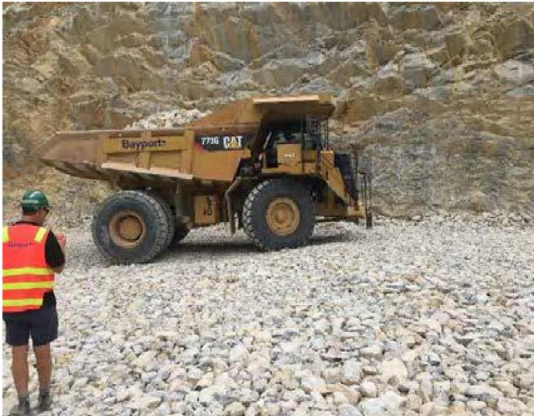
**Figure 3 showing the gravel drainage blanket in the base of the quarry.**
