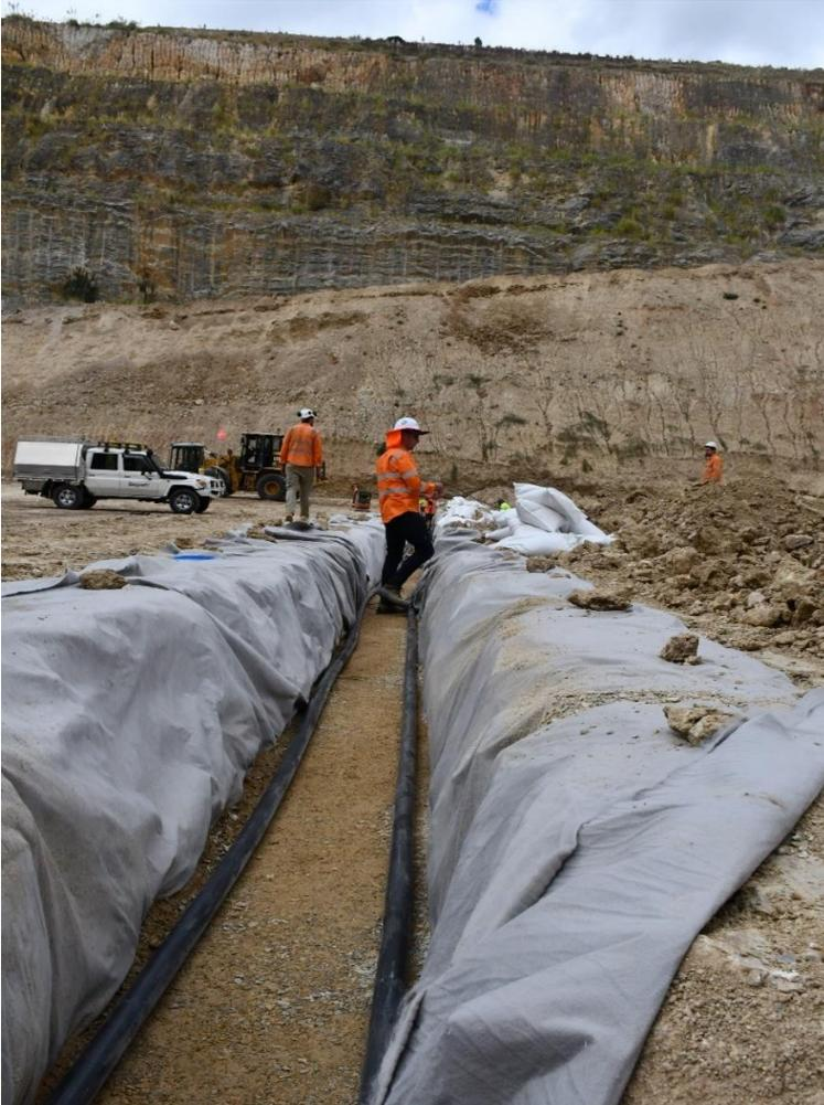
**Figure 6 showing typical installation of settlement and piezometer array.**
